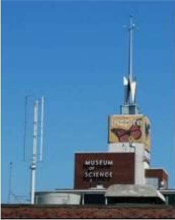
(LEFT) Shown here on the Blue Wing roof, Windspire Energy's 1.2 kW @ 13m/s vertical-axis turbine is 7 meters high, including the 4 meter rotor. This Extreme Wind model replaced the Standard model in July 2011.
