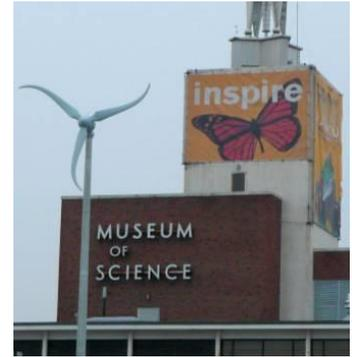
(RIGHT) Southwest Windpower's Skystream 3.7, also on the Blue Wing roof, is a downwind, horizontal-axis 2.4 kW @ 13m/s design with a rotor diameter of 3.7 meters, mounted on a 10 meter tower.
