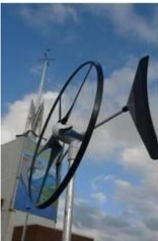
(LEFT) The Swift, manufactured in the U.S. by Cascade Engineering, is a 1.0 kW @ 11m/s, upwind, horizontal axis design with a 2.1 meter diameter. It features unique rotor and tail designs, and is mounted on the center building roof.
